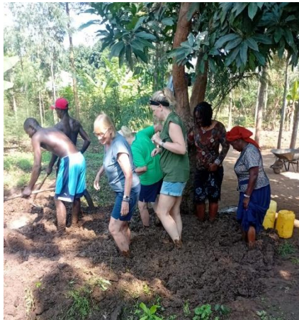
Mixing soil for mudding walls
