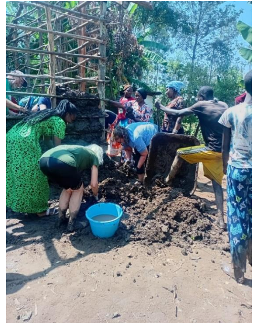
Putting mud on house side for walls
